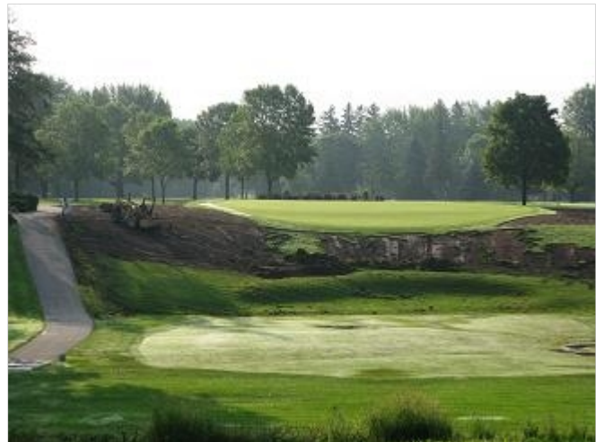
2) Beginning Reconstruction Work
